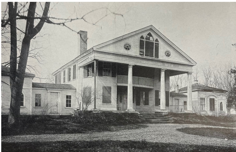
Vaucluse, front (south) view
